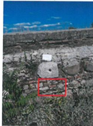
Aq-4: masonry mortar from the lower part of the pillar, inner layer.
