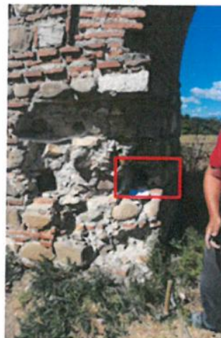
Aq-4: masonry mortar from the lower part of the pillar, inner layer.
